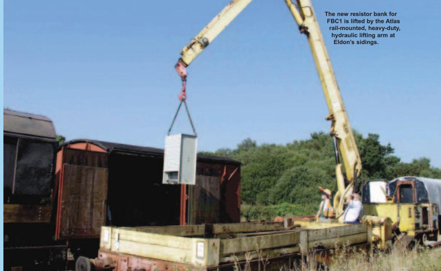
The new resistor bank for FBC1 is lifted by the Atlas rail-mounted, heavy-duty, hydraulic lifting arm at Eldon's sidings.
